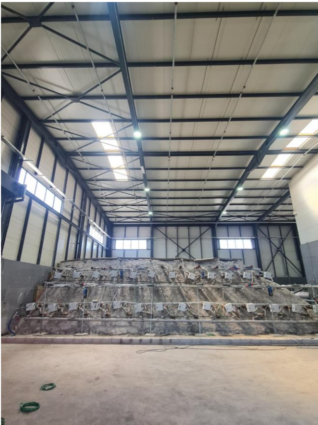
Figure 1. Pile 600t in Ritsona, Greece
